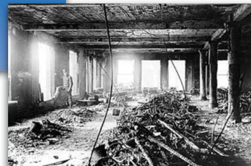
After the fire, devastation.
